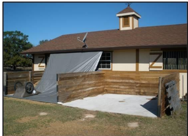
Ideal AFO manure containment system built on a family farm with 8-12 horses on the property. Photo credit: Jamie Cohen.
