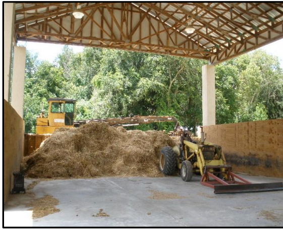
Ideal CAFO manure containment system taken at a CAFO racehorse facility in Ocala, FL. Photo credit: Jamie Cohen
